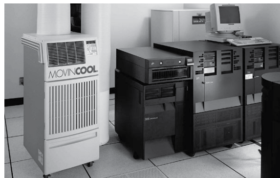
Portable air conditioner with condenser plenum and two ducts creates a closed-loop system for efficient after-hours server room cooling
